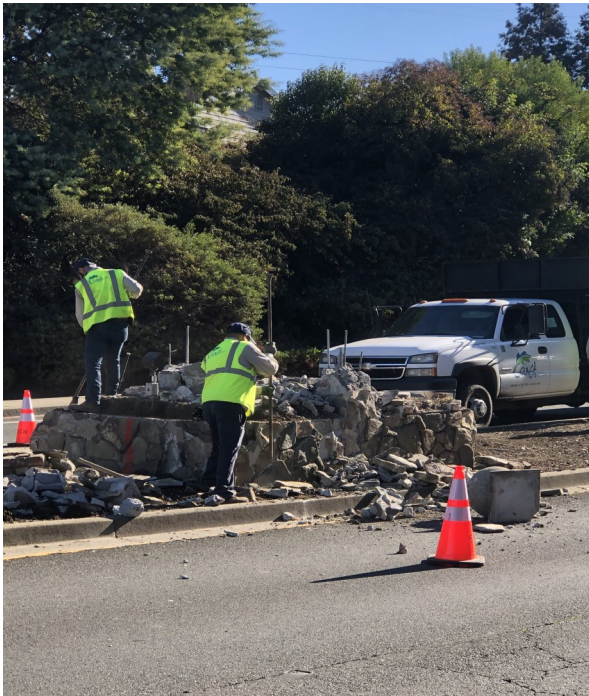
LMD crews removing the old monument (Picture by Ward Stewart)
