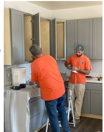
Fire house renovations in progress
